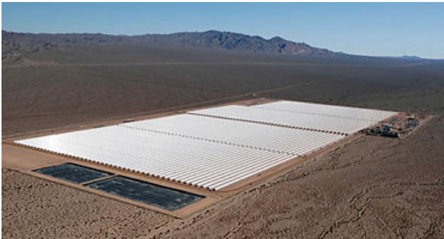
Fig. 2.16 Nevada Solar One CSP plant
